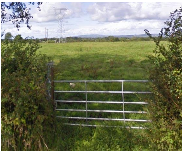
Existing entrance at Coole for Mountphilips Substation
