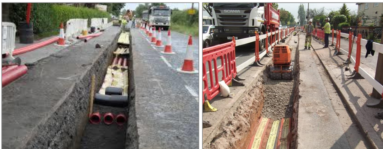
Plate Error! No text of specified style in document.2: Examples of underground cable trench in public road
