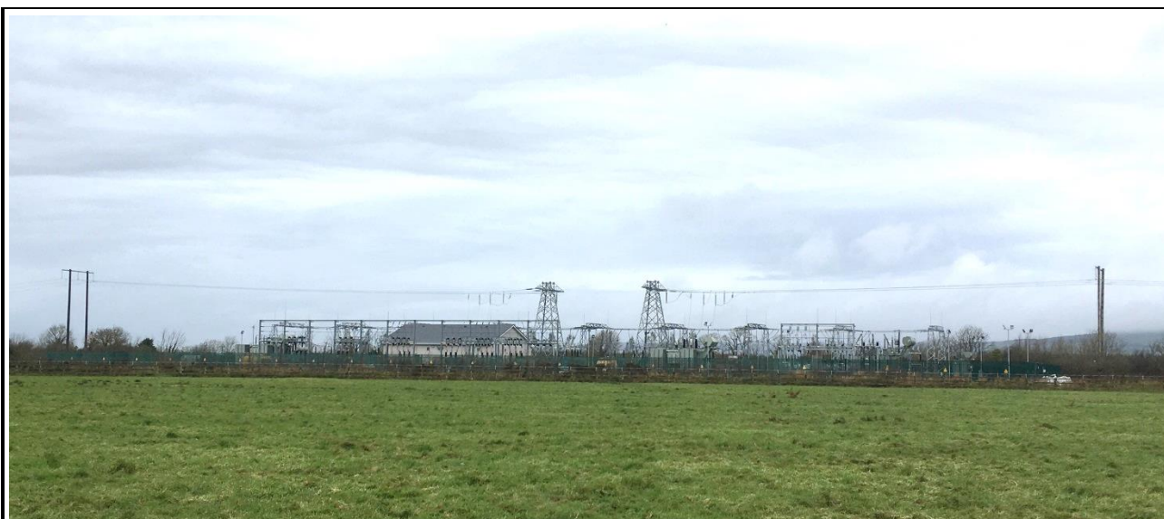
Example of similar 110kV substation with End Masts connecting to overhead 110kV line
