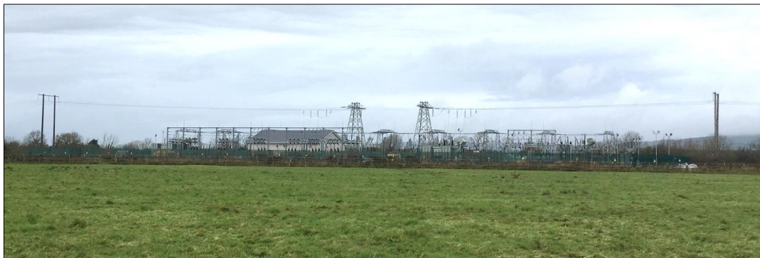
Plate 1: Example of similar 110kV substation with End Masts connecting to overhead 110kV line
